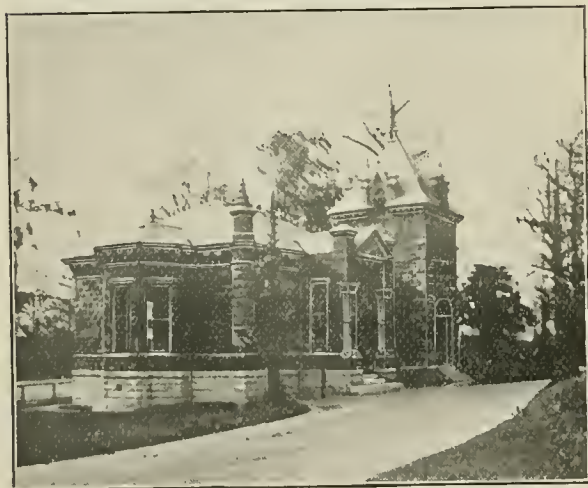
LODGE AT ENTRANCE OF OAKDALE CEMETERY, WILMINGTON.
